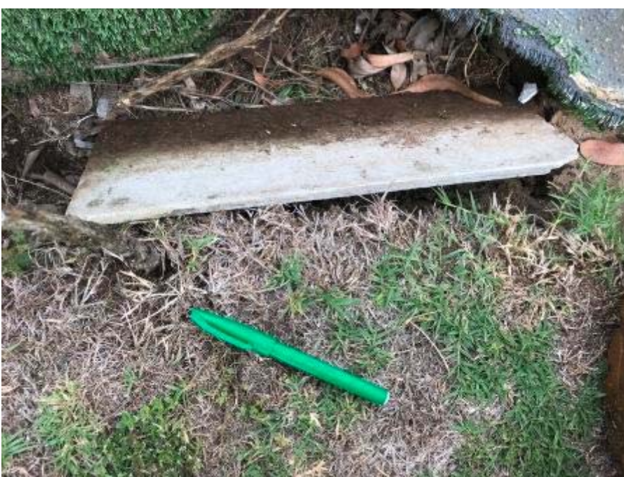
Image 6.10.4 View of fibrous cement sheeting along edge of bowling green
